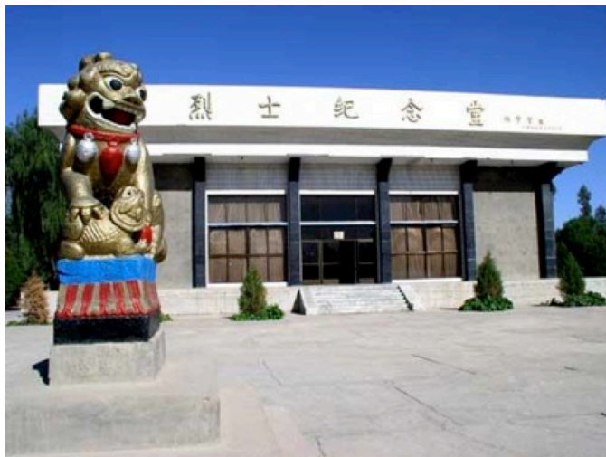
Fig. 7-5 The museum in Gaotai Cemetery for Martyrs before renovation (from Gansu National Defense Online, downloaded on July 24, 2015).
